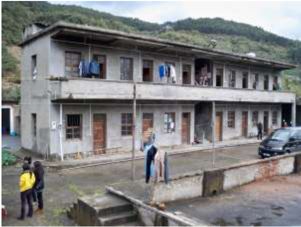
The new residential program under renovation, located on a fish farm.
